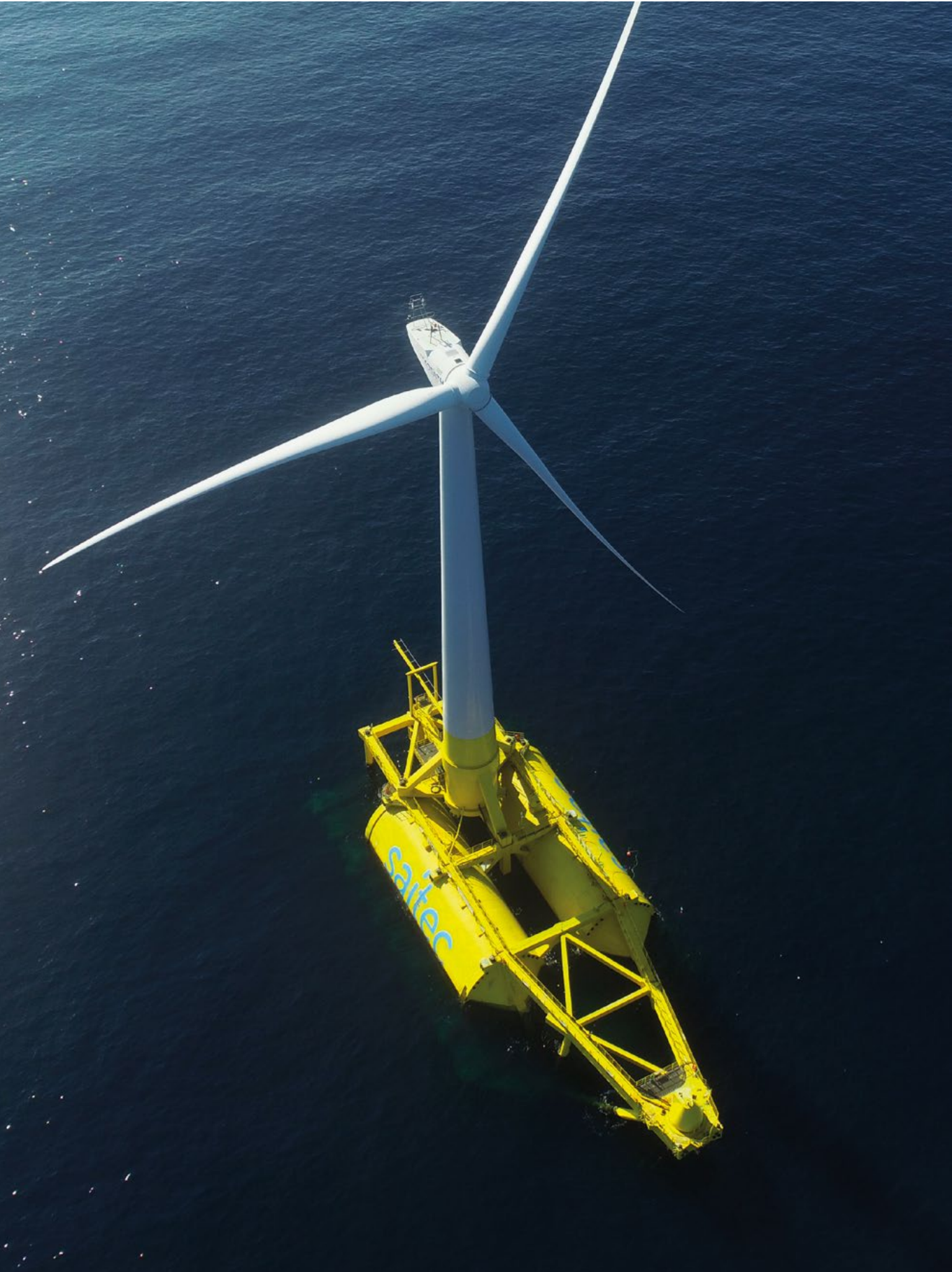
FLOATING DEVICE INSTALLED AT BIMEP
