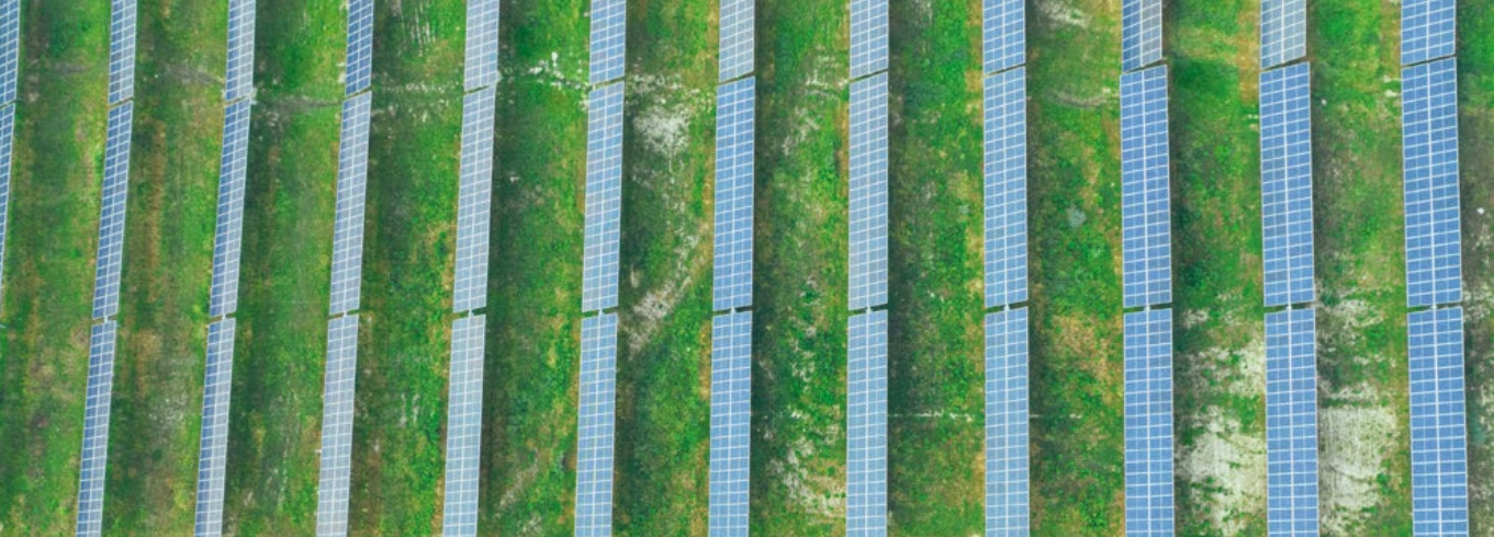
AERIAL VIEW OF EKIAN SOLAR FARM
